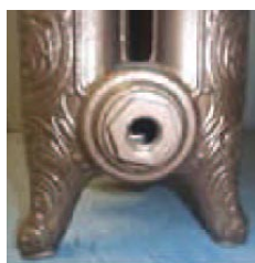
Two 1/2" BSP threaded bushes for the connection of radiator valves
